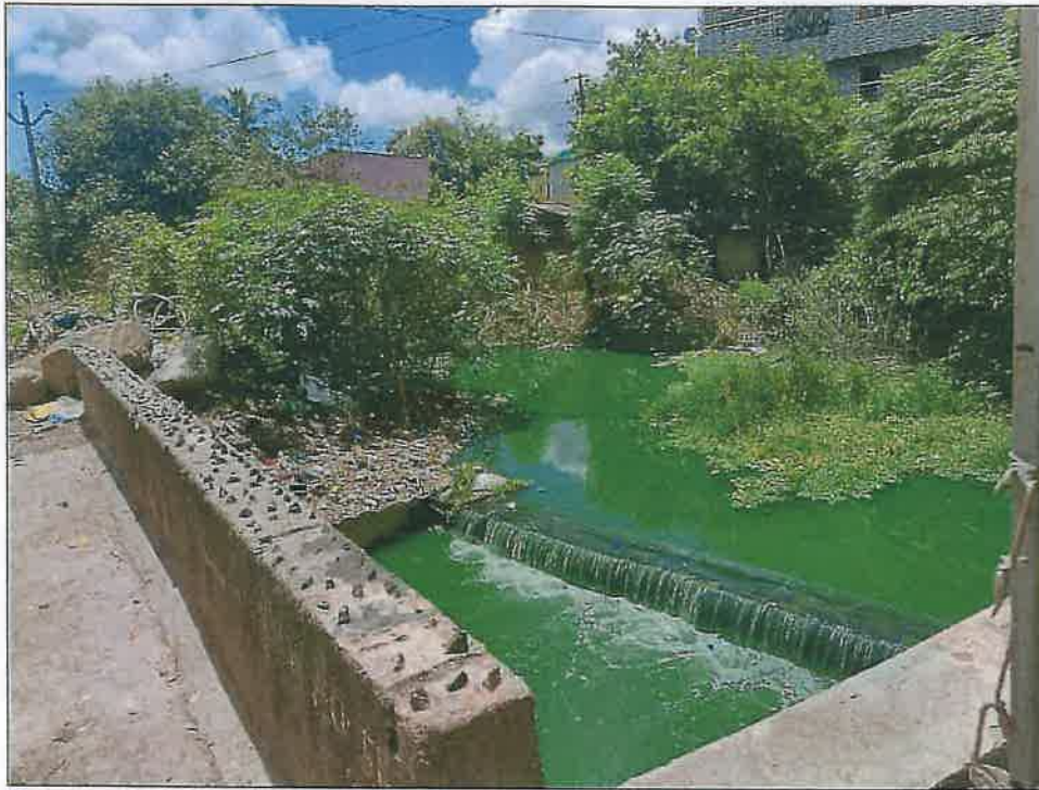
KADAPPERI LAKE overflow line into MEPZ (PIC 3)
